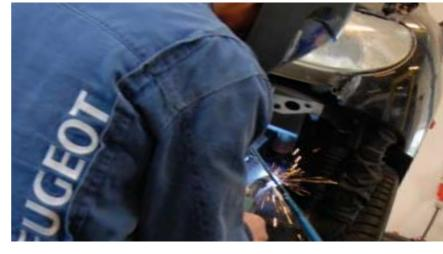
MIG brazing is used on a large scale for the construction of car bodies and other transport vehicles in galvanised high tensile steel to maintain strength properties in the steel and to protect the anti-rust zinc coating.
